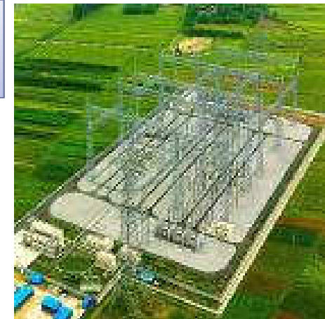
Nanyang Power Transmission Facility
